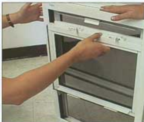
Swing other side into alignment with the jamb.
