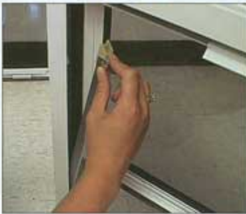
Hook the balance terminal clip into position, slide balance down and secure top guide under the take-out clip.
