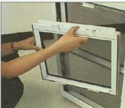
Insert one side of the vent into jamb 2" - 3" above the take-out clip.
