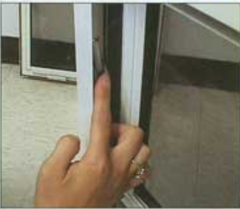
Install take-out clips, upper and lower, and leave in open position.
