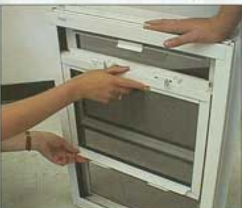
Lowering vent to engage balances and clear take-out clips will automatically center it.
