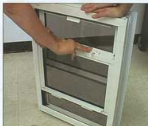
Close vent and fasten check rail latch. To remove vents, reverse the installation procedure.
