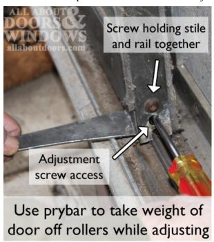
**14.** Check operation of door, making sure lock functions correctly (lock on sliding panel lines up with strike on frame). Adjust until door is in correct position.
